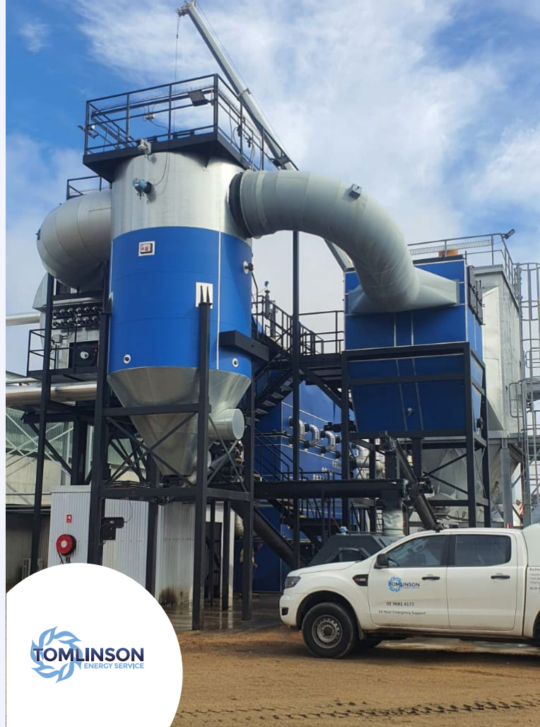
12 MW Biomass Heating High Temperature Hot Water Boiler, Dongwha NSW
