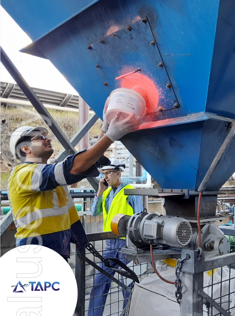
TAPC Bag Filter Service: Visolite Leak Detection Test, Pt Kembla, NSW
