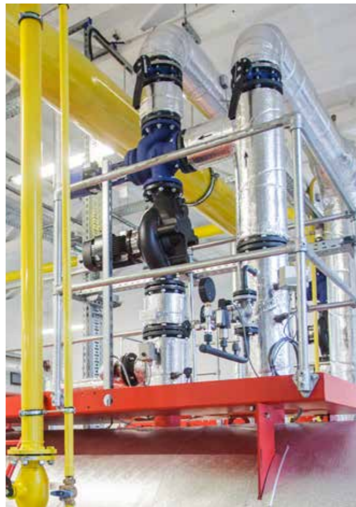
Return flow temperature safeguard RTS
