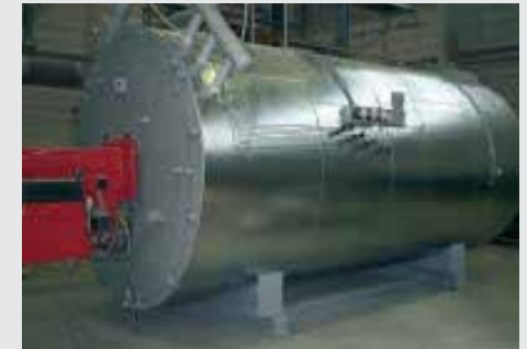
Thermal oil heater fired with natural gas with a capacity of 1.6 MW, installed in Texas, USA, application in the food industry
