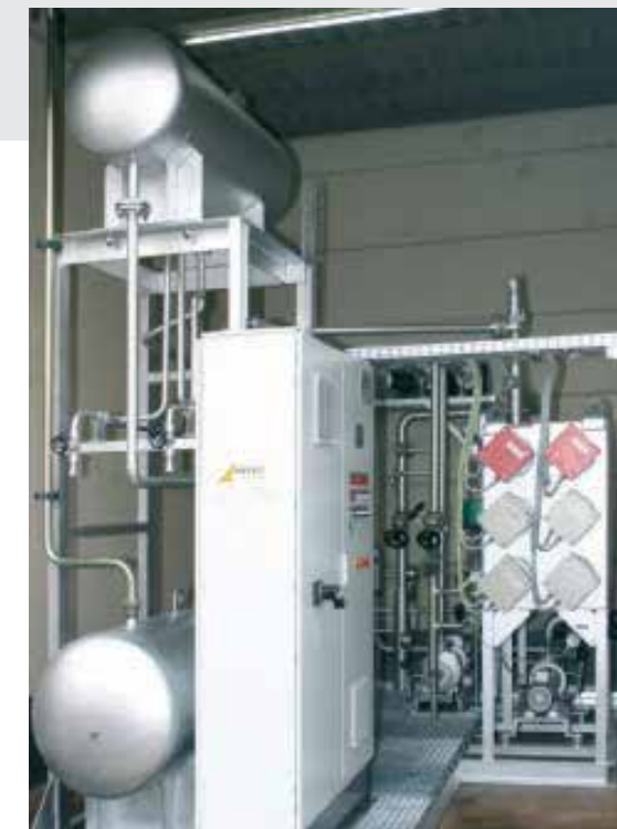
Electric heater with an output of 150 kW with six heating elements for exact regulation of capacity
