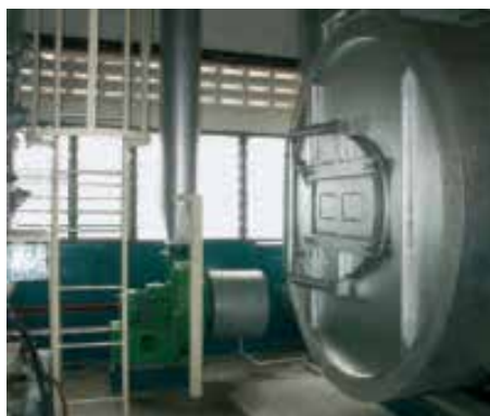
Horizontal heater with a net capacity of 10 MW with combustion air preheater, access door at the reserving chamber for the inspection of the combustion area (Malaysia)
