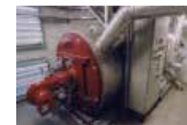
Horizontal heater for the food industry, premounted and wired as compact unit
